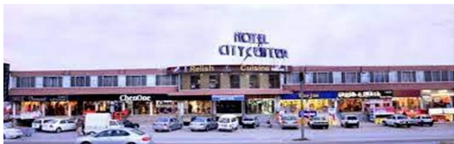
Figure 20 City Center Front view
